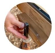
There is a locking device to ensure the slide is locked into place. Turn this lock once slide is in position.
