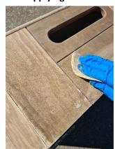
1) Wearing gloves, apply the oil liberally with a rag or large paintbrush. Rub excess off with a clean rag after 1-2 mins ensuring to wipe along the grain.
